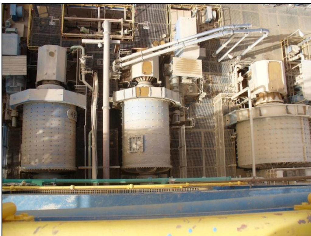
Figure 40: Overhead View of SAG and Ball Mills
