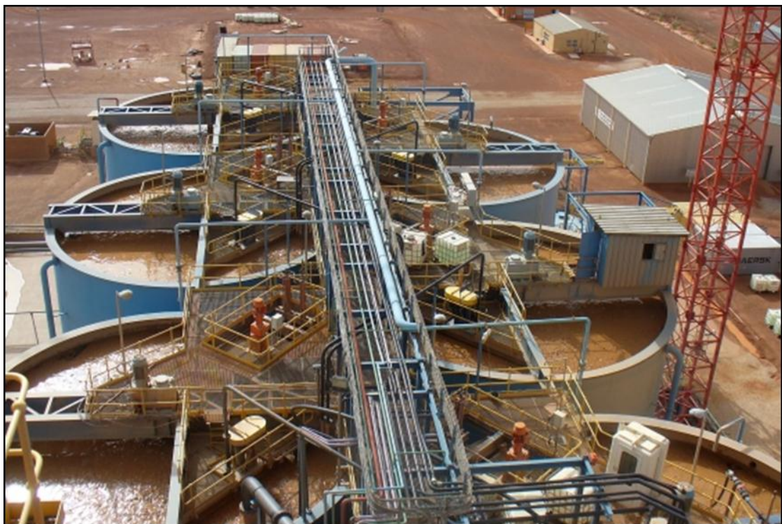
Figure 42: Process Plant CIL Train
