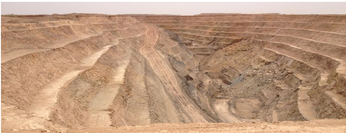
Figure 23: Photo of Central Pit looking north
