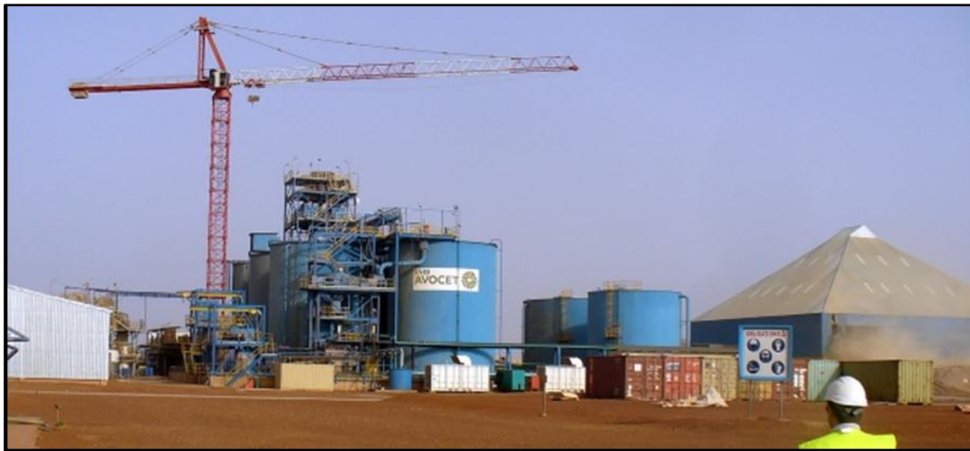
Figure 17: Inata Treatment Plant
