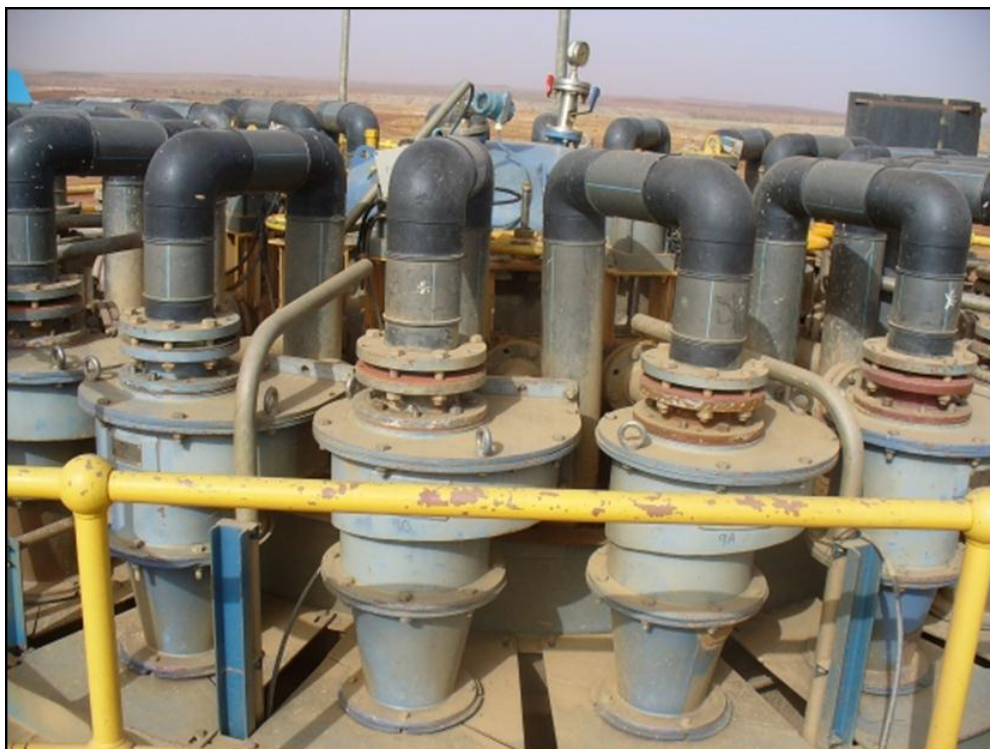
Figure 41: Grinding Circuit Classification Cyclones
