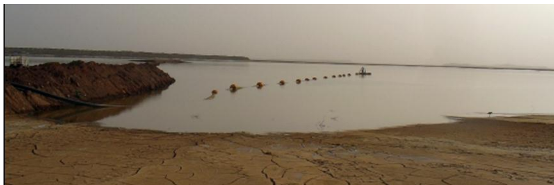
Figure 46: Existing Tailing Storage Facility
