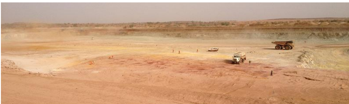
Figure 27: Minfo Pit looking south
