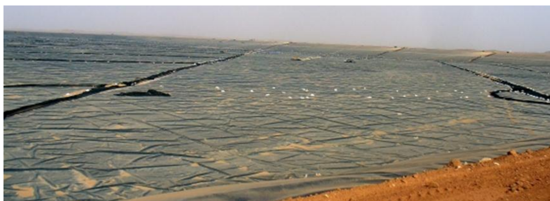
Figure 47: Newly Constructed Tailing Storage Facility (TSF 2)
